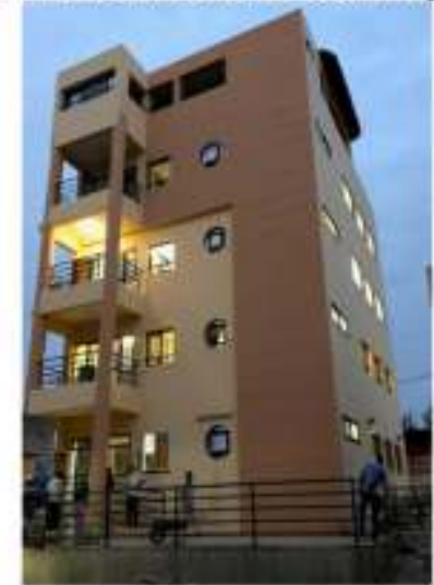
DELGEME Permanent training facility
